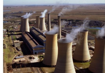
FIGURE 3: VIEW OF KOMATI POWER STATION
